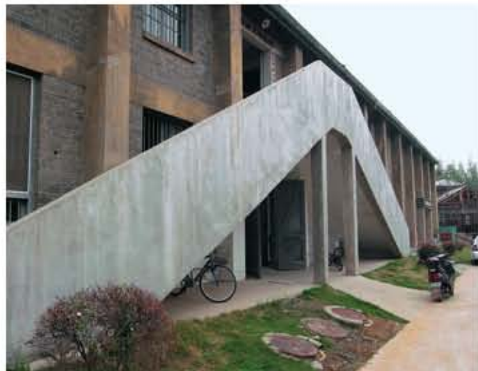
南京一处改造后的工业建筑 Former industrial site refurbishment, Nanjing
